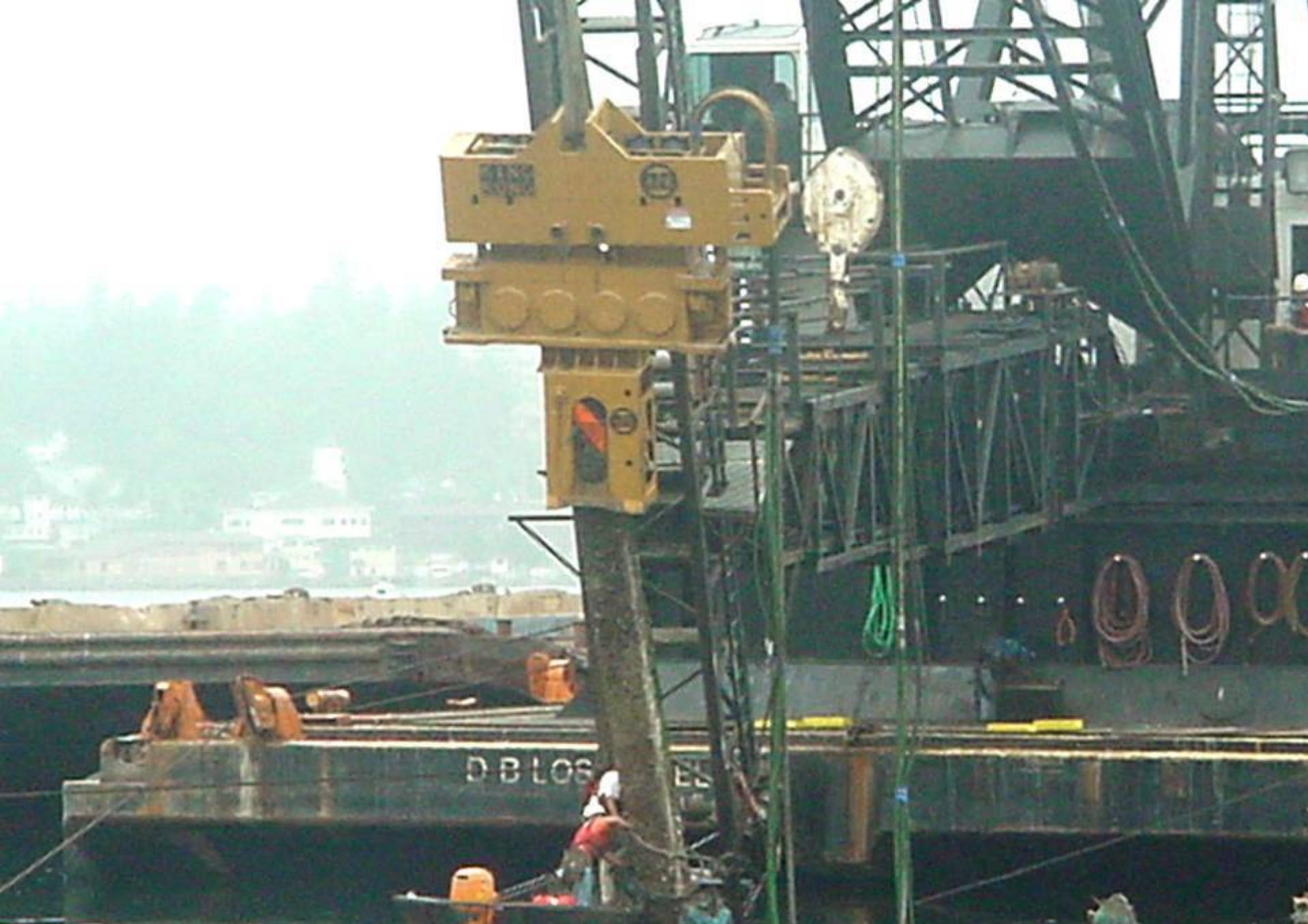
APE Model 400 in leads extracting Concrete Piles
