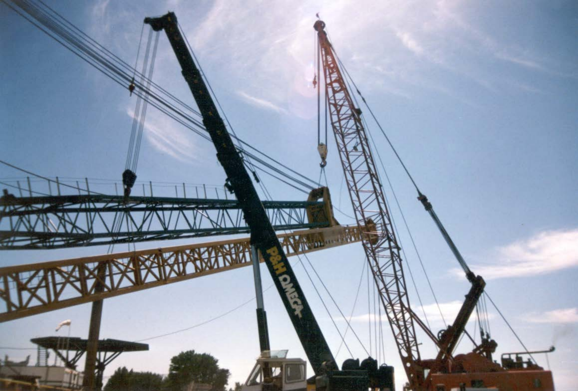
Two cranes help assist piling crane in picking fixed lead system
